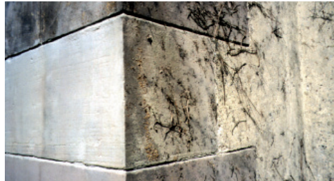
Stonewall before and after cleaning
