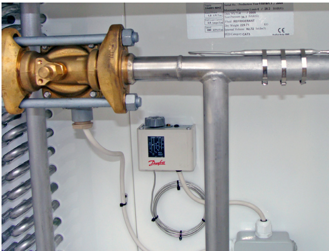
1'000 kg/h (2'204.62 lb/h) atmospheric ASCO CO 2 Vaporiser: Thermostat
